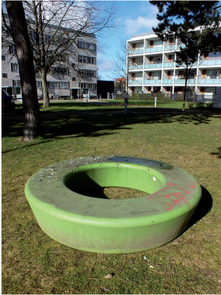
1: Before cleaning (LOOP from a Copenhagen park, 7 years old when these photos were taken).
